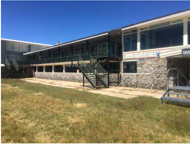
Figure 3: Photo of the northern side of the hotel and staircase to be replaced and airlock to be constructed
